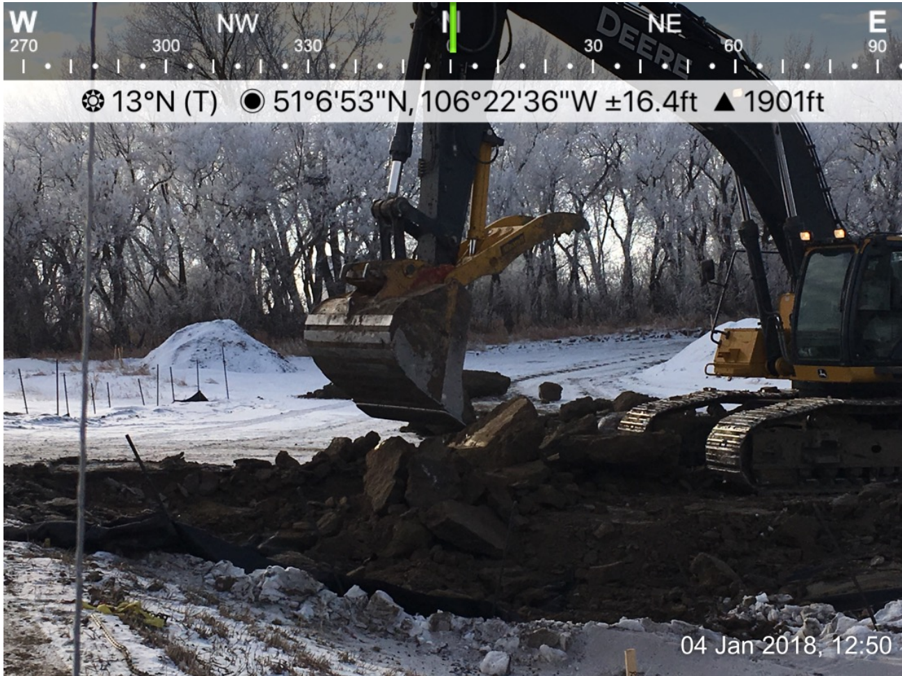
CLEANING UP OF TOPSOIL OFF APPROACHES
