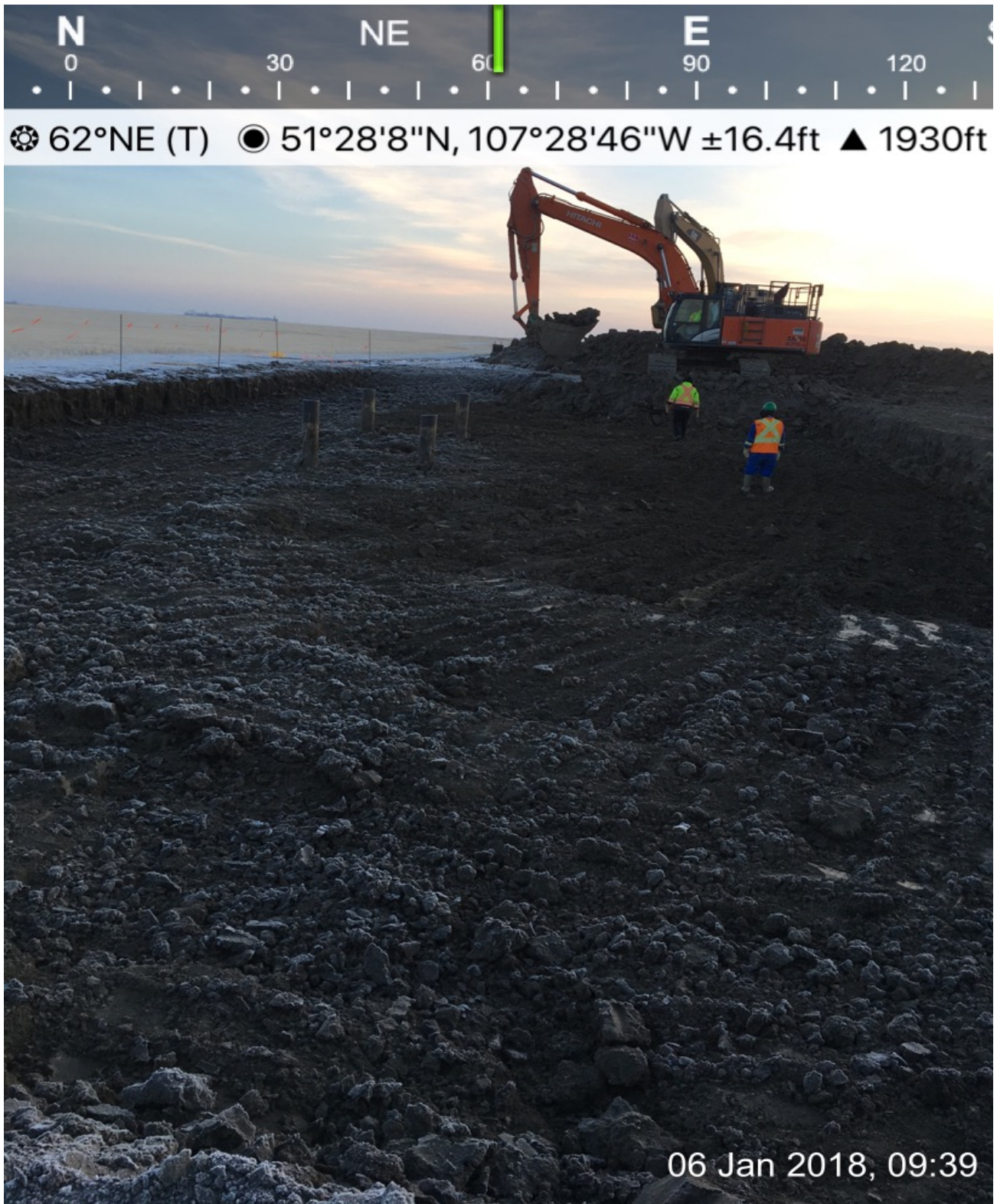
EXCAVATING WHERE VALVE IS GOING TO SIT
