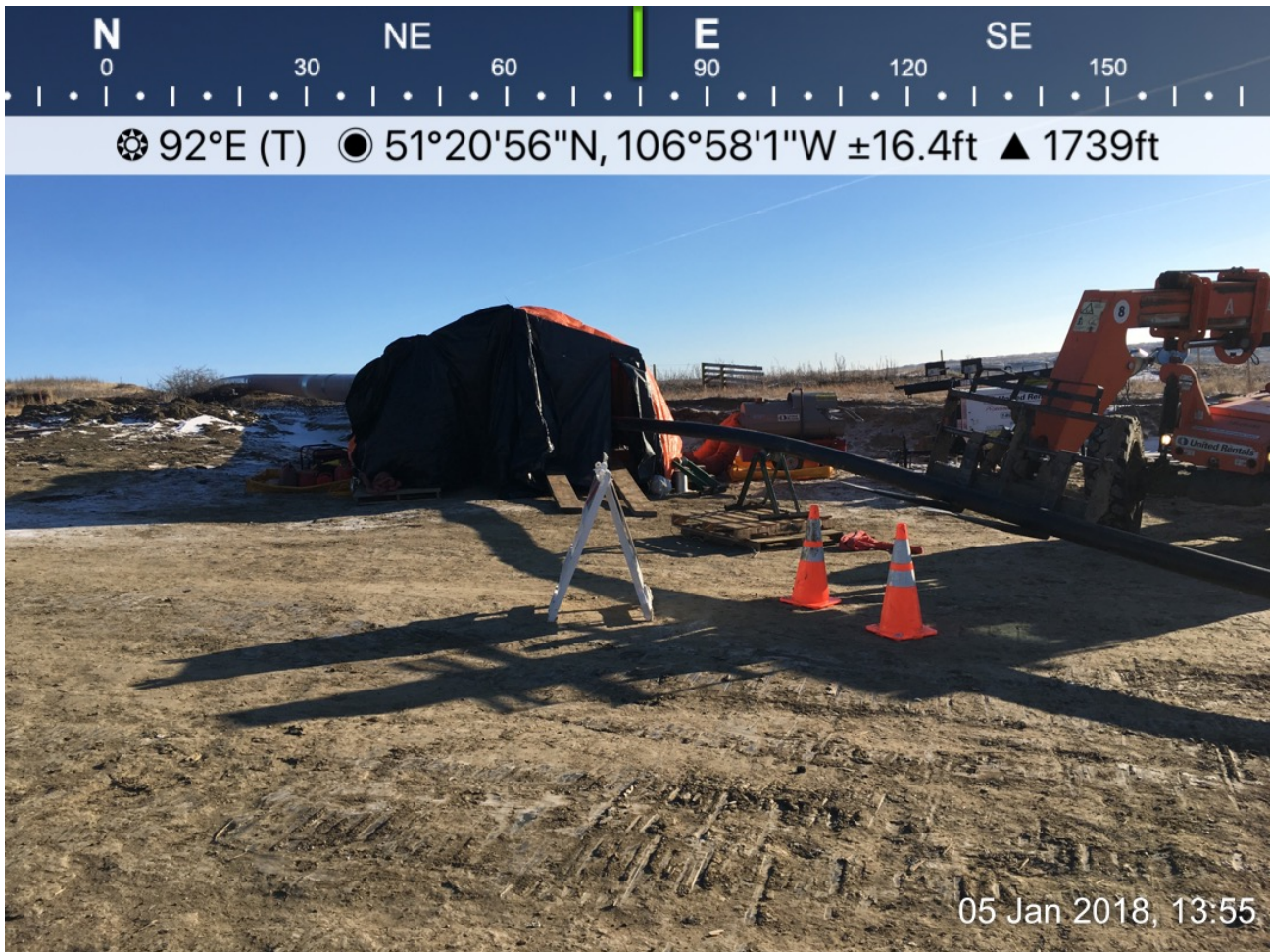
INSTALLING BUOYANCY PIPE IN BORE SECTION
